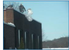
fall hazard. The first person up the ladder should observe the rung conditions, clear off snow, and use a hammer to knock any ice off the rungs.
